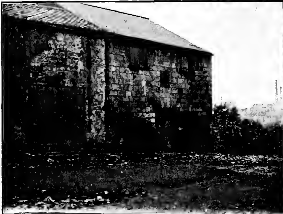
TADCASTER FIRST CHAPEL. End building, Rosemary Row.
