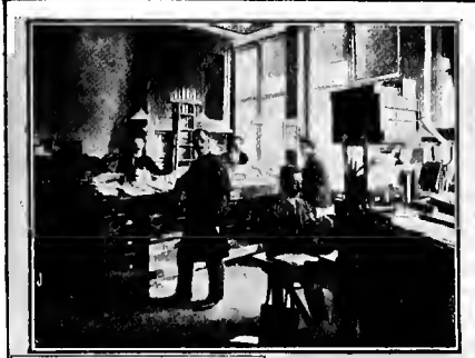
THE GENERAL OFFICE AND PART OF THE OFFICE STAFF
